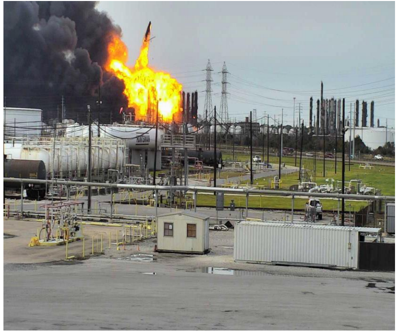
Figure 7. Explosion at 1:48 p.m. on November 27, 2019 which propelled one of the South Unit towers. (Credit: Huntsman Corporation)
