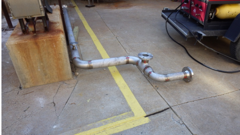
FIGURE 2. 20-foot replacement piping (Source: CSB).
